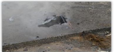
**4.2.1.2** Roof plates corroded to an average thickness of less than 0.09 inches in any 100 inch area or roof plates with any holes through the roof plate shall be repaired or replaced.
